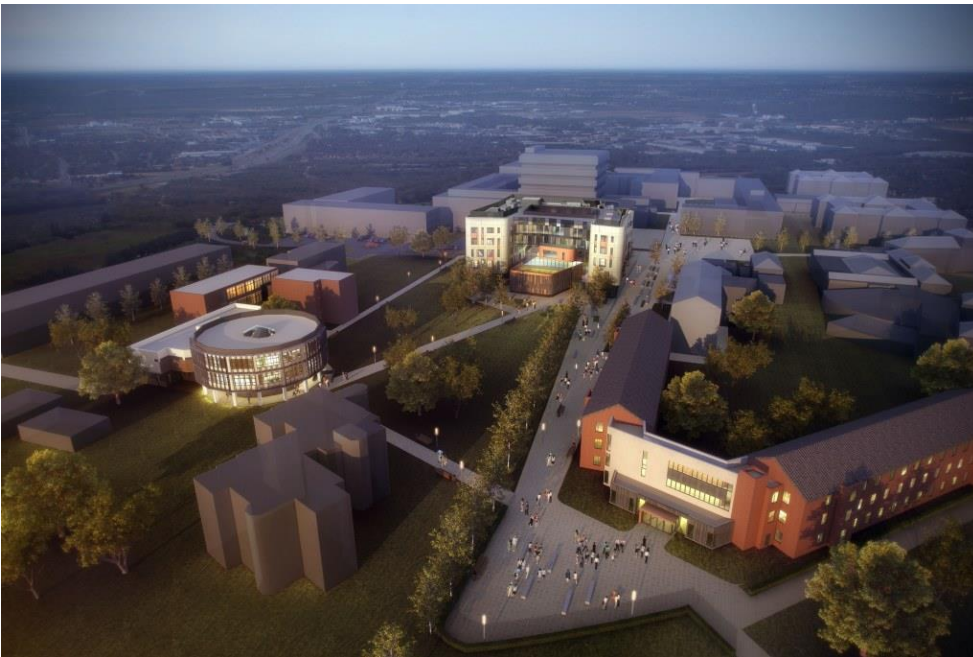
Aerial image of planned Health Campus development at University of Hull, due to open in June 2017.
